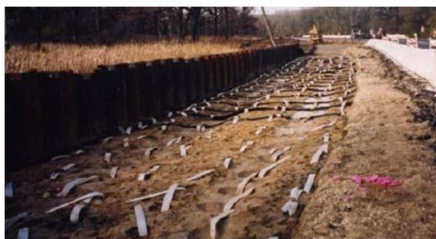
Figura 10 Geodreni verticali in opera
