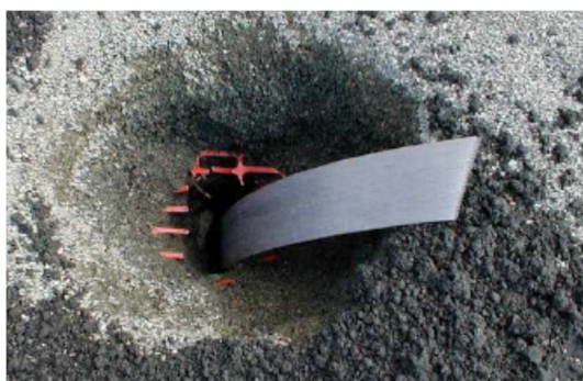
Figura 10 Geodreni verticali in opera
